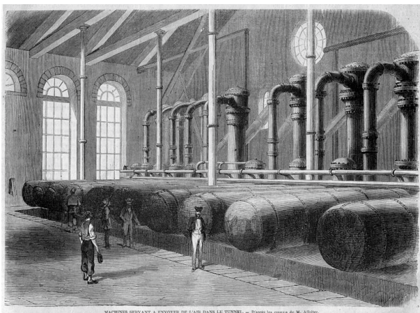
Serbatoi aria compressa From Wikimedia Commons, the free media repository
