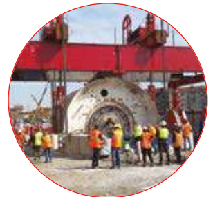
416 ton: Transport, Lowering and Installation
