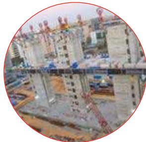
Installation of 10 complete Floor Slabs : Strand Jacks
