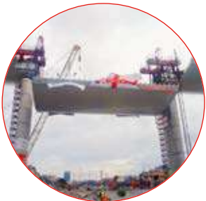
Installation of sections weighing up to 2,000 ton
