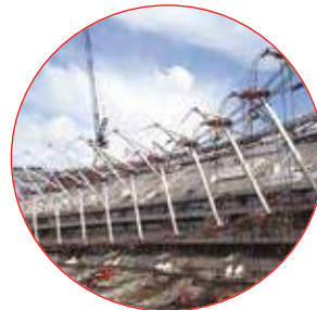
216 Strand Jacks working simultaneously
